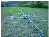
Assemble the antennas onto the mast, the blue work stool playing its part in providing some working space under the masting pipe.
