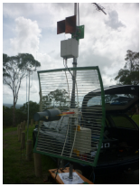
View from the other side of the antenna array...
