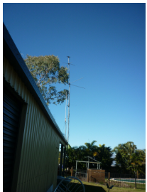
Better view of the antennas..
