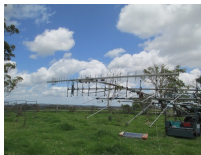
VHF/UHF antennas - phase 2 - with the 23cm yagi on the top.
