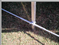
The U clamp bolts through the element & around the boom
